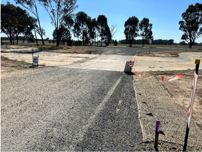
Photo 7: Hardstand stabilised site access, main compound
