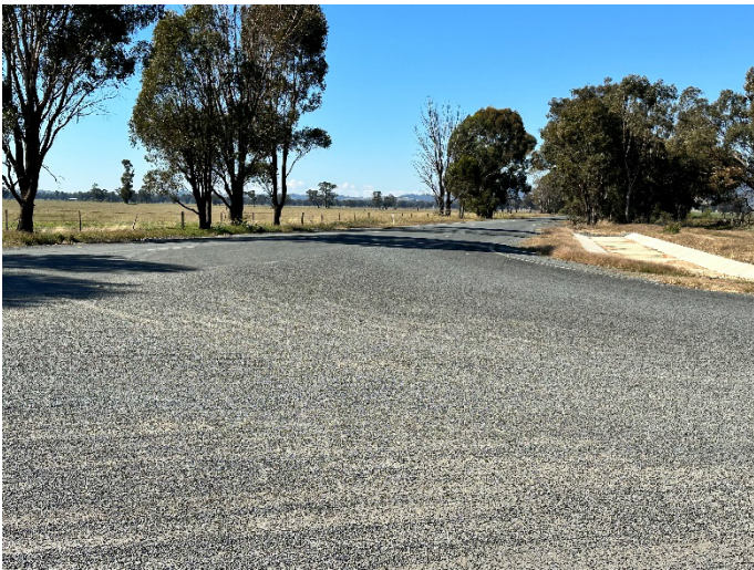
Photo 3: Upgraded intersection with Benambra Road
