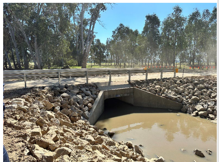
Photo 12: Permanent culvert drainage and scour protection
