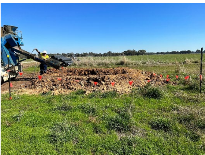
Photo 11: Concrete washout pit
