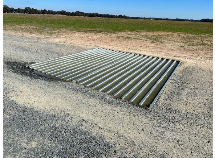
Photo 8: Rumble grid at main site compound exit point
