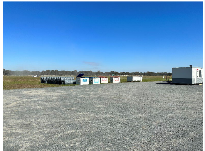
Photo 10: Hardstand site compound and waste storage bins
