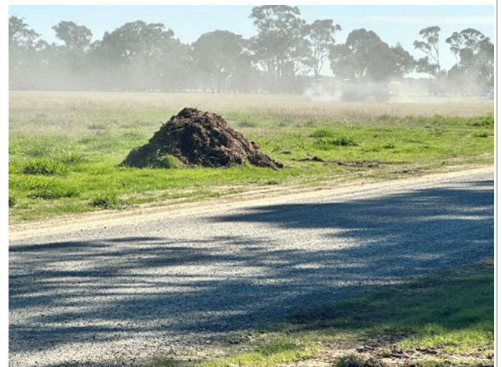
Photo 18: Mulch stockpile, located away from drainage lines
