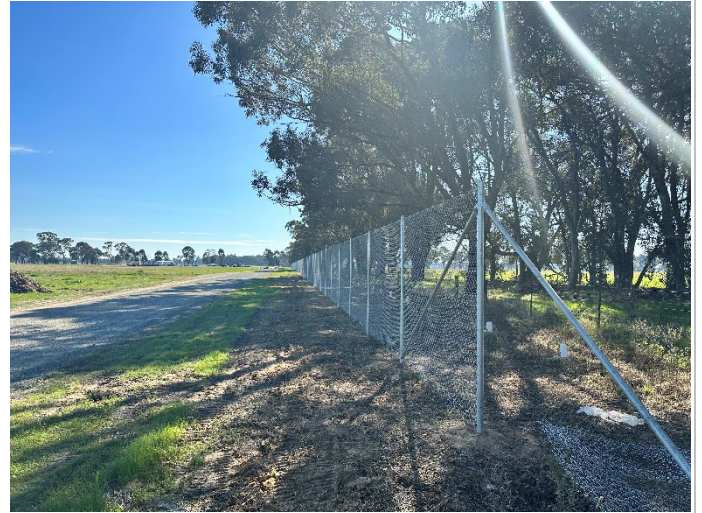
Photo 2: Permanent site boundary chain wire fencing
