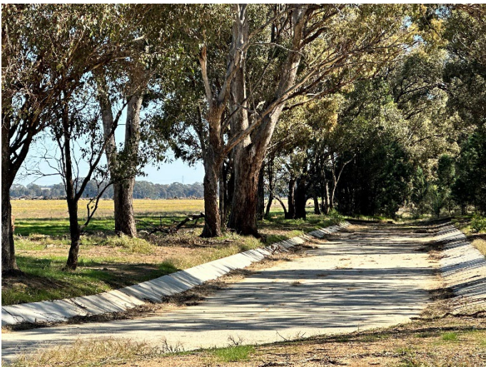
Photo 5: Permanent perimeter drainage
