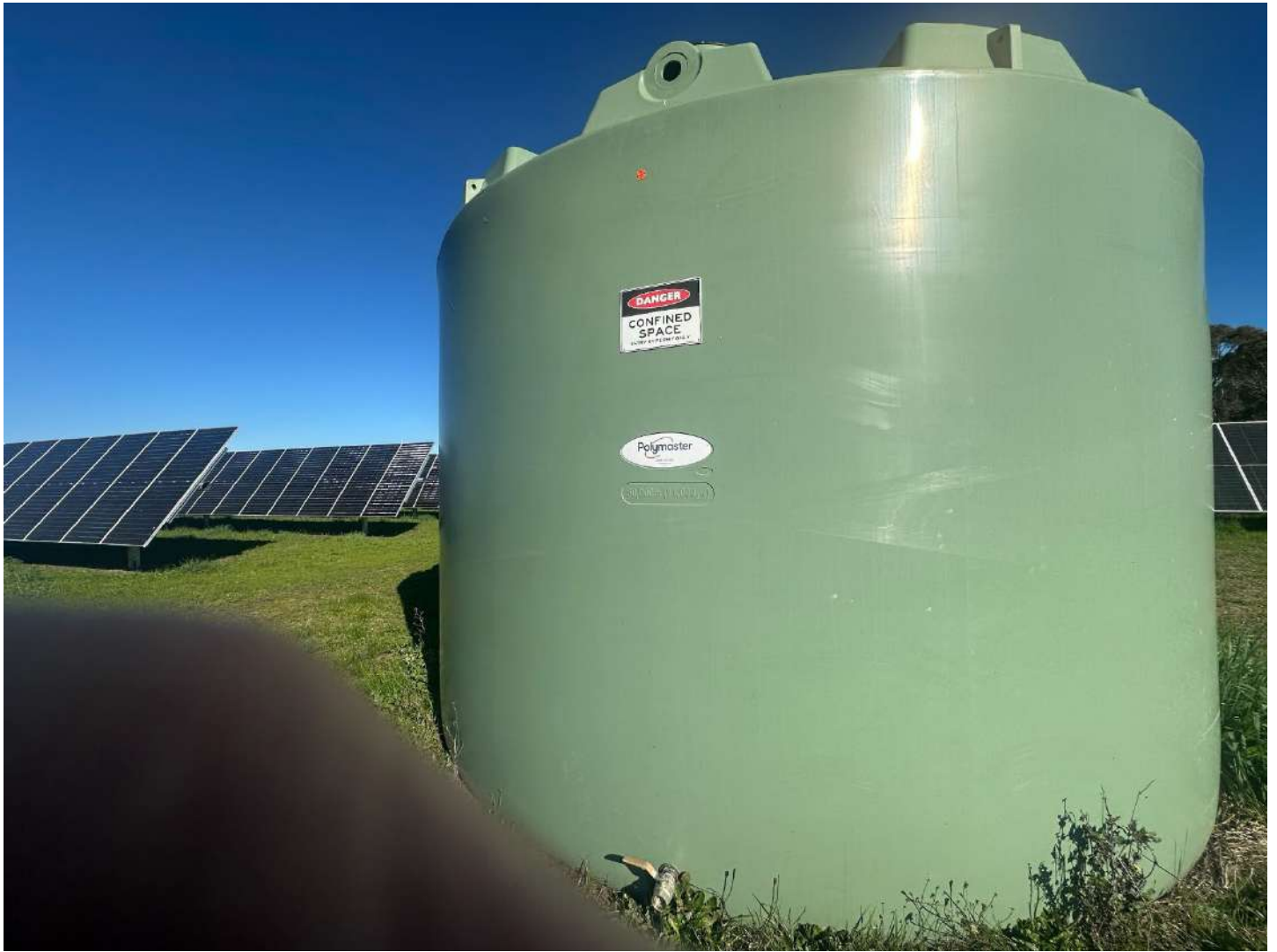
Photo 19: 50,000L fire water tank
