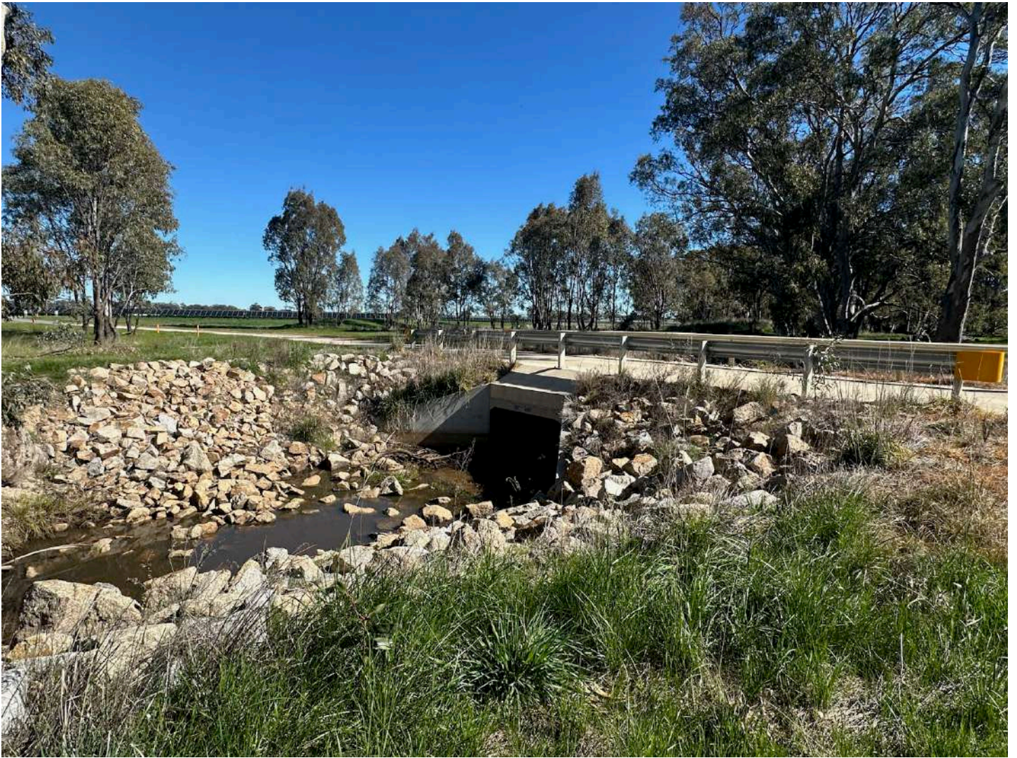
Photo 23 – permanent stormwater culvert and rock scour protection
