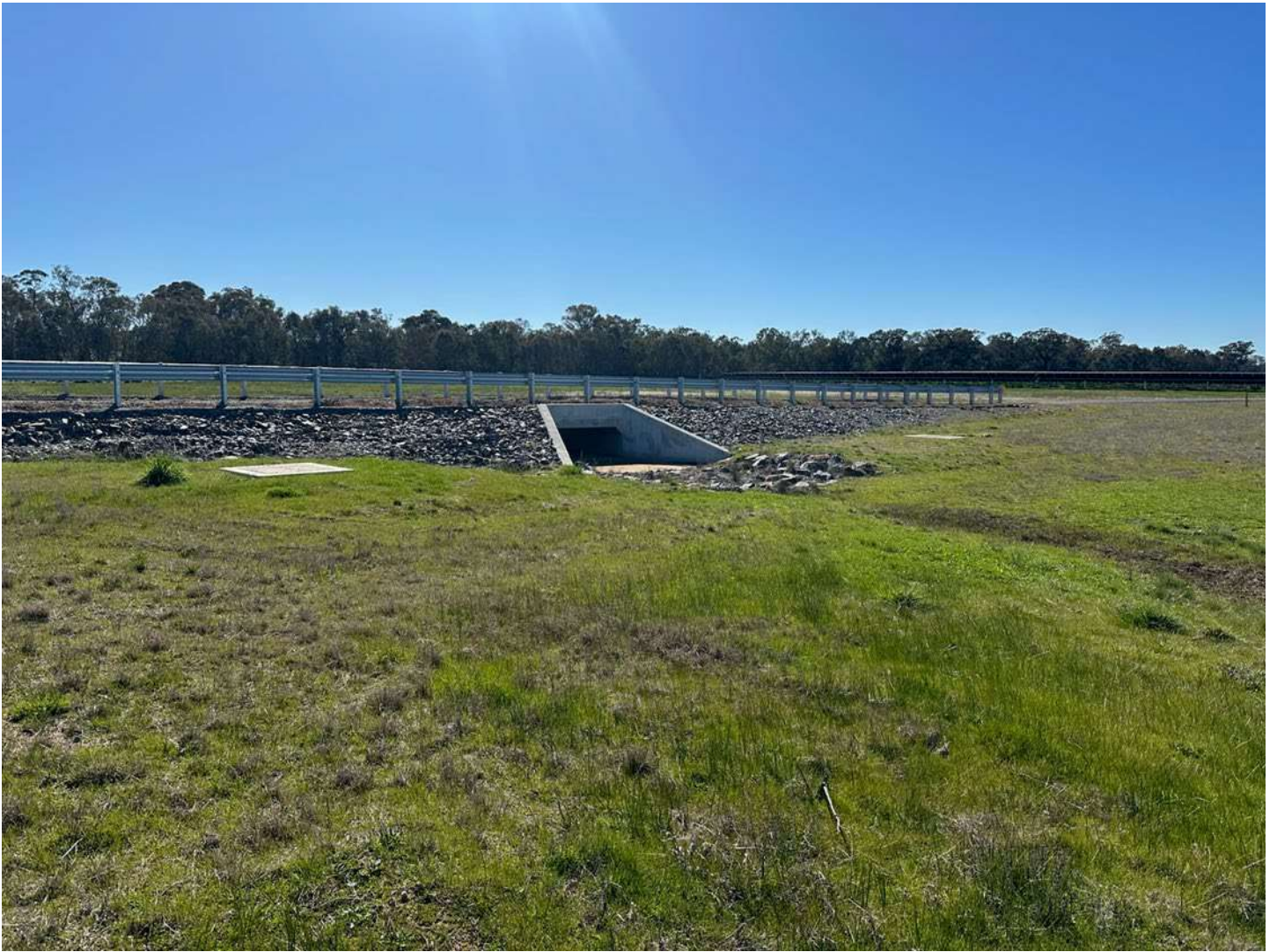
Photo 24 — permanent stormwater culvert and rock scour protection
